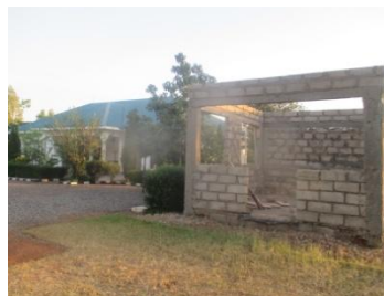
The waiting area under construction.
